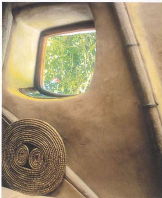
A section of the strawbale-sized walls (above)
