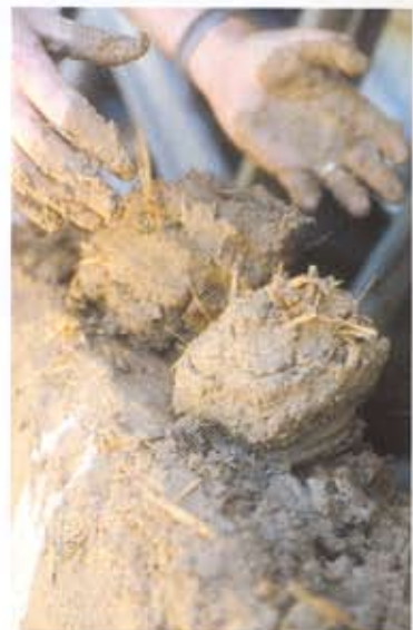
A cob ball, made of straw and clay, lands in the hands of the builder (right) after having been passed down the line like a rugby ball
