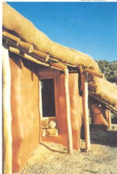
ABOVE & LEFT: A completed house (bungalow) with its plastered straw bale roof and walls.
